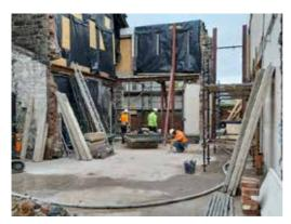
Currently the old link building has been demolished, except for the section that needs to be retained and this is currently being supported by a specially made support structure. The piling has been completed, also the foundations have been dug out, the sub structure drainage and concrete sub floor has also been completed.
