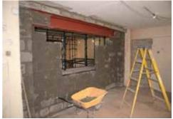
The wall between the hall and kitchen has been removed and rebuilt as a thinner section with a larger service hatch and our kitchen supplier will now be coming out to take their final measurements so we can then put the plans in place to get the new kitchen installed.
